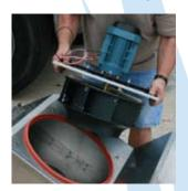
The unique design of the IPVB makes is extremely easy to service if it ever becomes necessary. The entire drive unit can be removed without disconnecting the fan from the chimney stack system.
